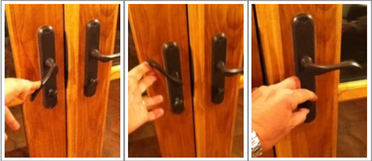
(from left to right) Pushing the handle down to unlock the door. Pushing the handle up to latch the door. Rotating the inside lock knob counter-clockwise to lock.
