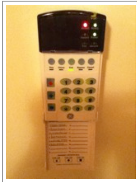
Alarm control pad. Exit button has been pushed and the red Armed light is on.
