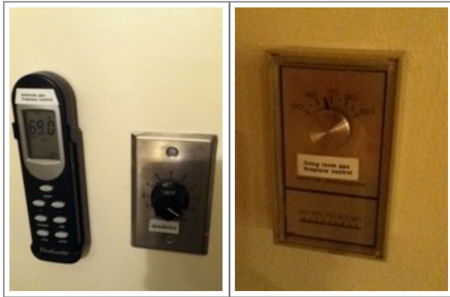
(left) Thermostat control for the bedroom fireplace next to the volume control for the wired speaker system in the bedroom. Shown on the display is the current temperature and the fact it is in “auto” mode. The top button in the on/off button . The two below it are the + and - buttons. (right) Thermostat control for the main fireplace.
